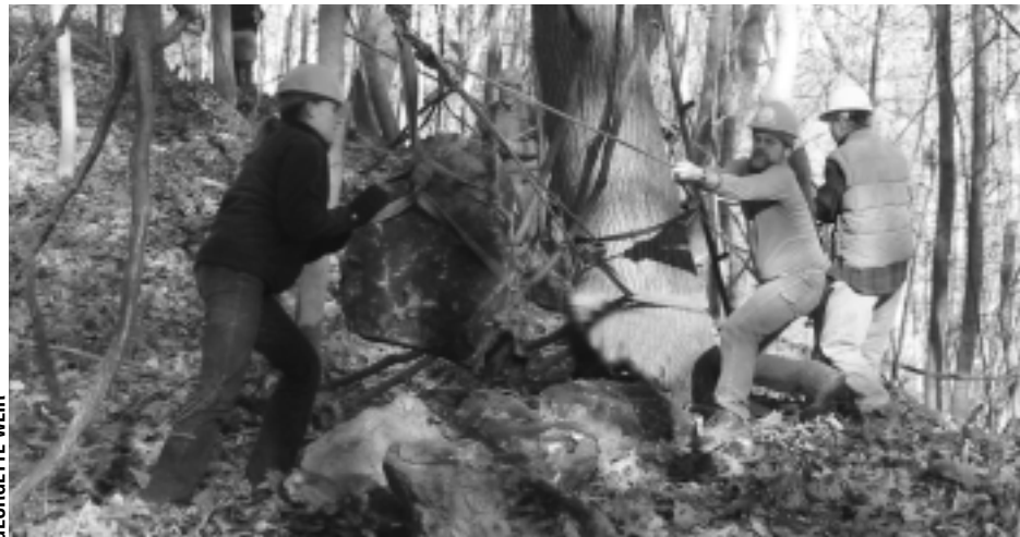
Kelly Dugan pushes a future rock step, Dave Webber pulls it, Denise Vitale secures the line, and crew chief Eddie Walsh (center, behind tree) works the winch.
