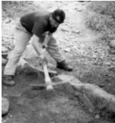
Bob Sickley repairs a waterbar on the AT to Sunfish Pond.
